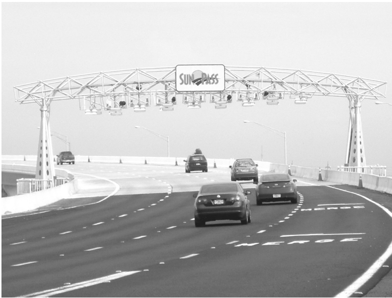
Fig. 2. Electronic tolling structure (gantry) collects tolls at free traffic flow speeds.
