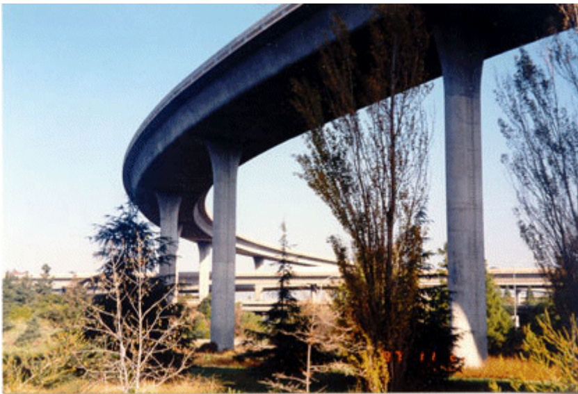
Fig. 3 Concrete girder bridge.
