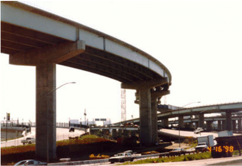
Fig. 2 Steel girder bridge.
